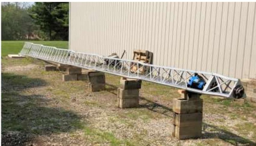
I also cleaned and started putting together the Yagi antenna that goes on the tower. It is a Cushcraft X-7 with the X-740 add on. However, the elements are too long to assemble in the building before mounting it on the tower so that part of the assembly process must wait until the 18' boom is attached to the mast. The task I just completed before writing this was driving in an 8' ground rod next to the pad and connecting it to a tower leg.
